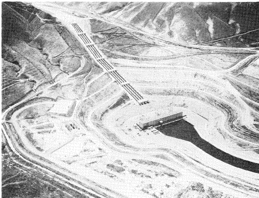
Pumping plants, such as the one shown above at Wind Gap, require significant amounts of electrical energy.
