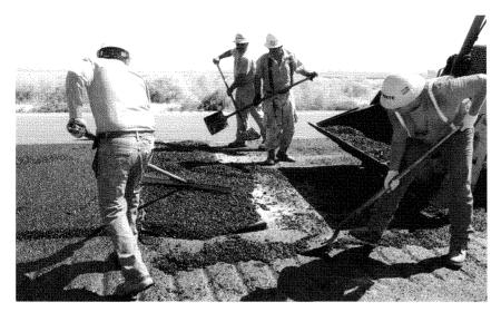
A rubberized asphalt operation on Interstate 5 in Fresno County.
