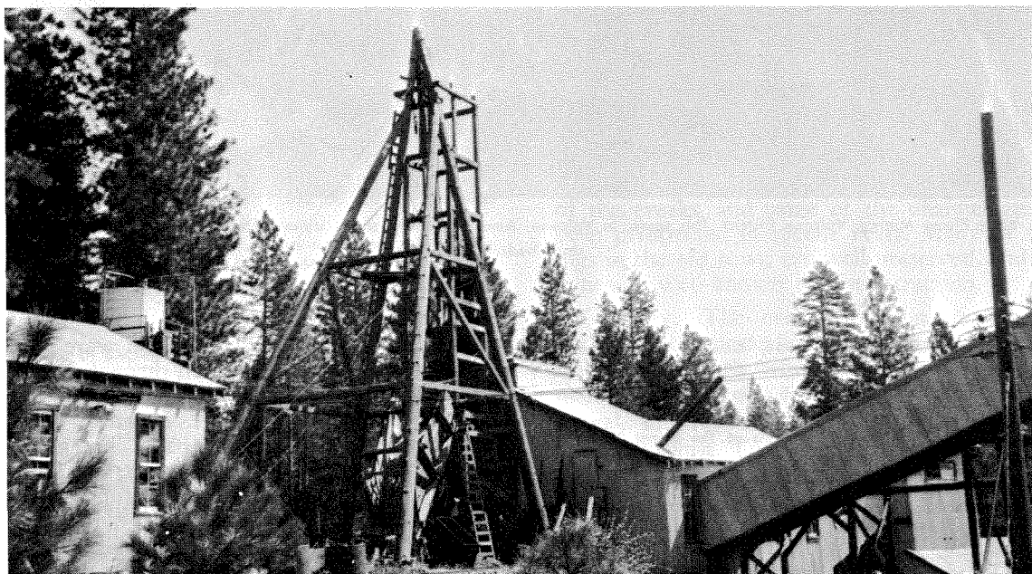
Photo 65. Belden Mine, West Point District. This 1952 view of the mine, in Amador County, looks northeast. The mine was active in the 1930s.
