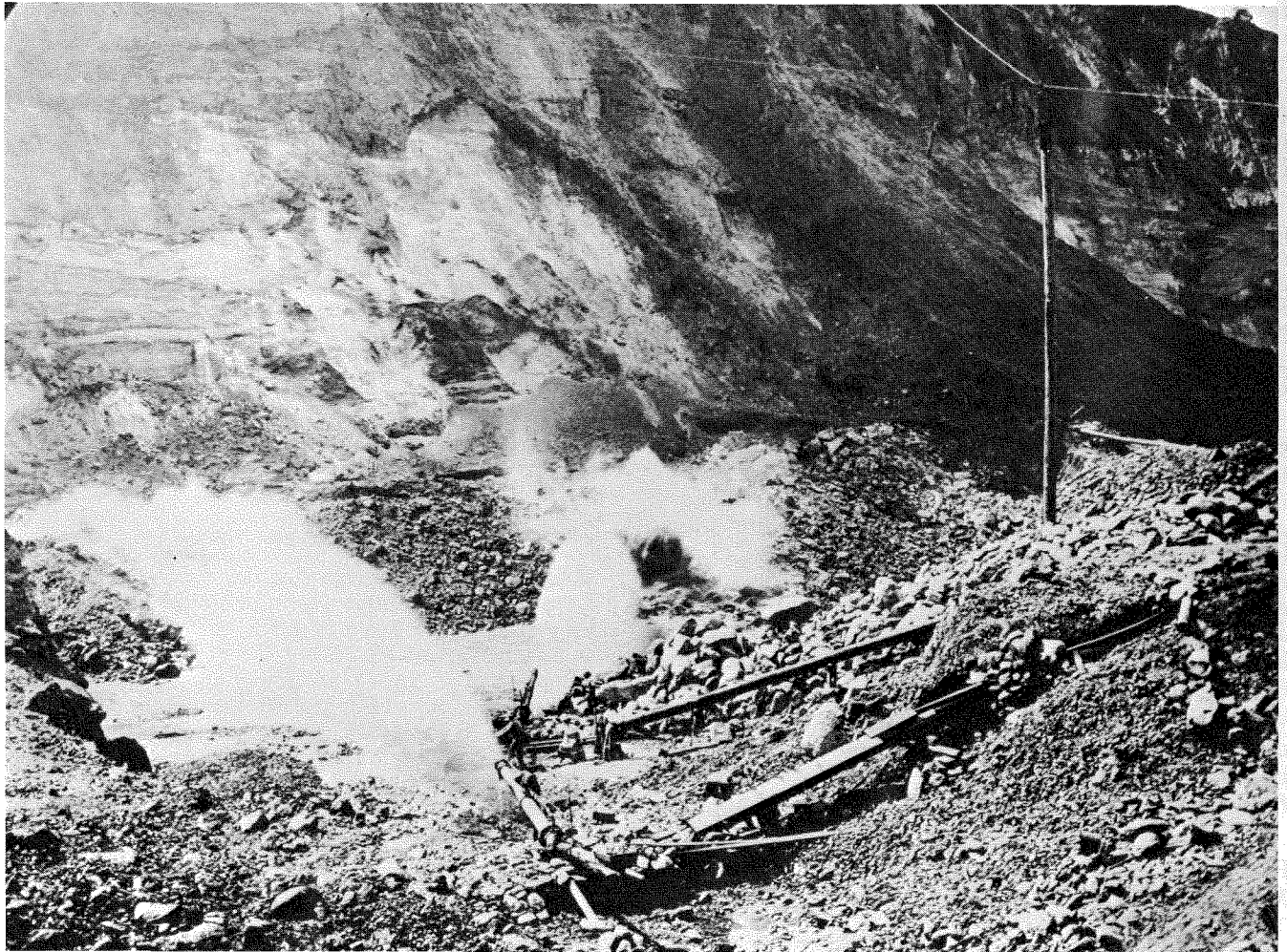
Photo 15. Cherokee Hydraulic Mine, Cherokee District. This view of the Butte County mine dates back probably to the 1870s. Photo courtesy of Calif. State Library.
