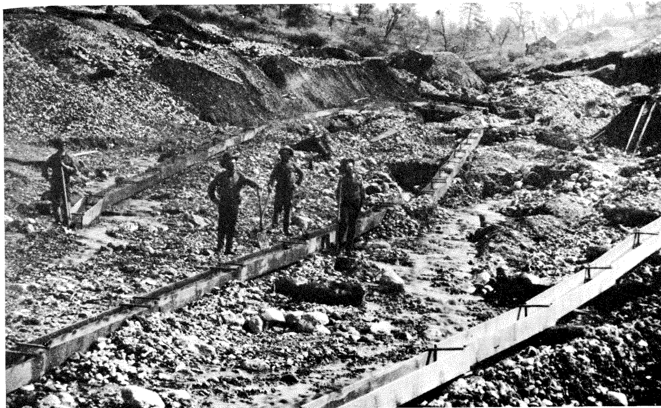
Photo 56. Ground Sluicing, Placerville District. This photo of an operation in the district, in El Dorado County, was taken in about 1849. From the collection of Mrs. T. J. Lobbard, San Francisco.
