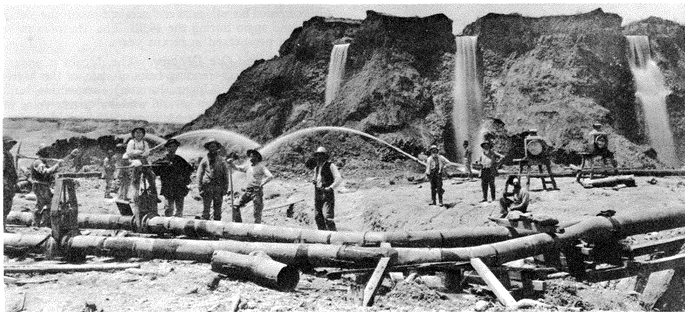
Photo 45. Hydraulic Mining in the 1860s, Michigan Bar District. This is a view of hydraulic mining and ground sluicing in Sacramento
