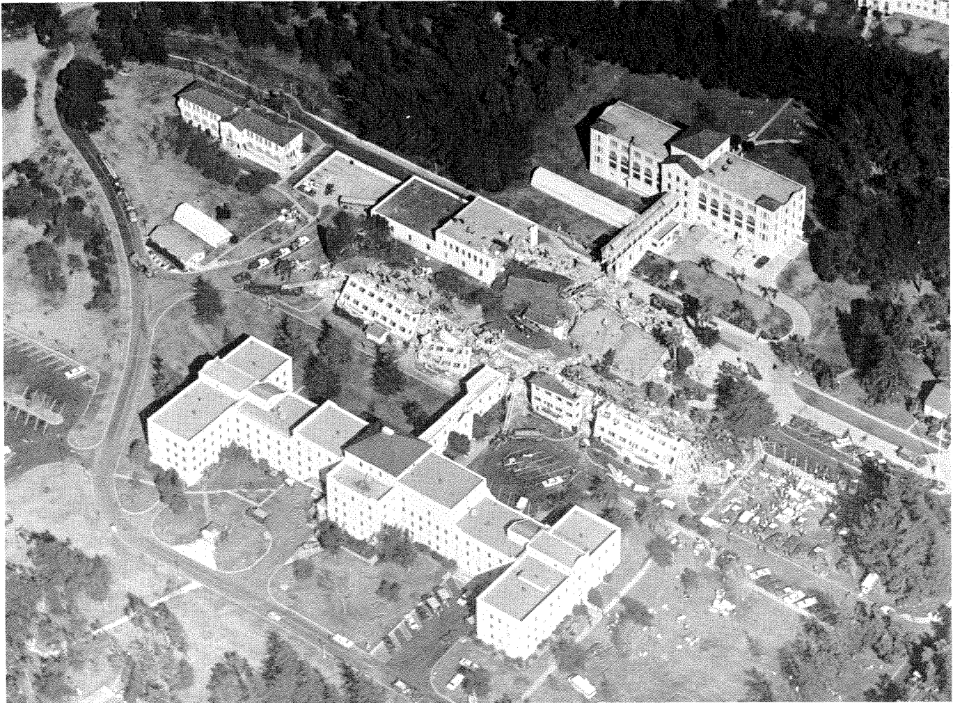
Photo 2. Aerial view of the damage at the Sylmar Veterans Administration Hospital caused by the February 9, 1971, San Fernando earthquake. Los Angeles Times photo.
