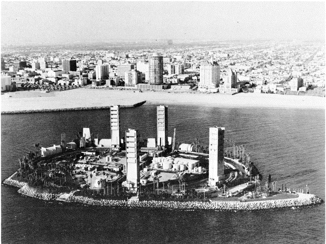
Photo 4. An artificial island near Long Beach used for petroleum production. Photo by City of Long Beach, Department of Oil Properties.
