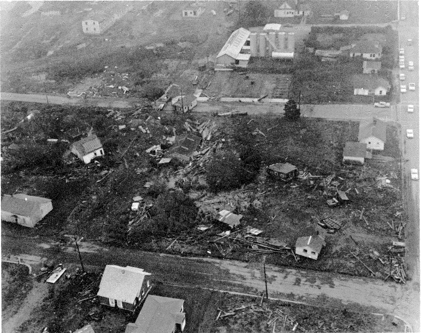
Photo 13. Tsunami damage at Crescent City, 1964. U.S. Army Corps of Engineers photo.
