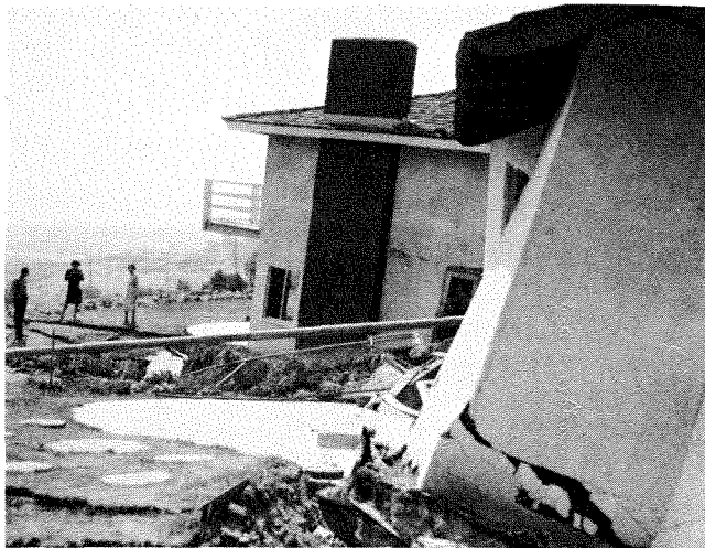
Photo 6. Homes destroyed by landsliding of artificial fill on the north slope of Palos Verdes Hills, Los Angeles County. Photo by George B. Cleveland.
