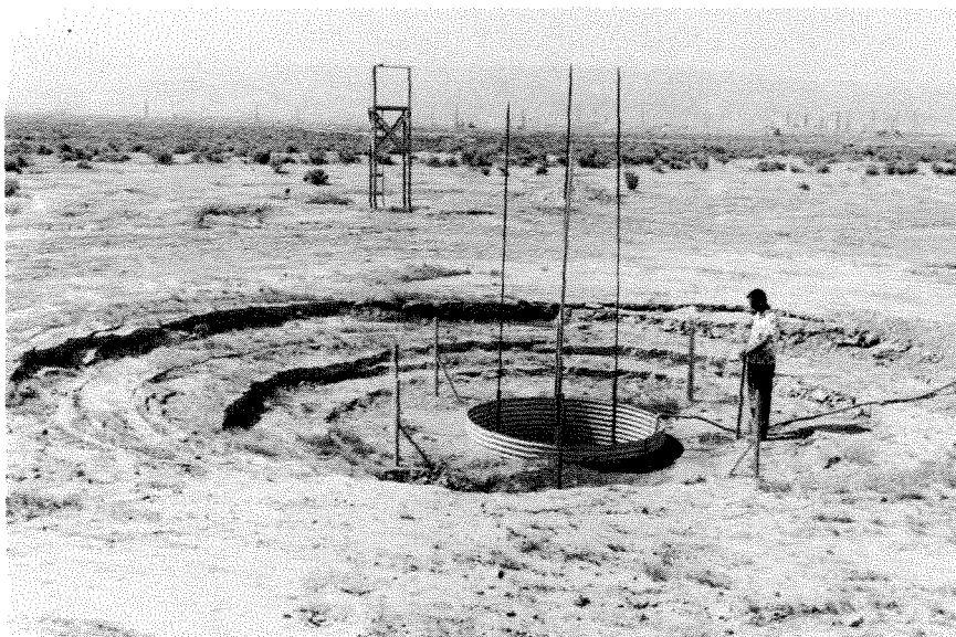
Photo 15. Hydrocompaction subsidence around a test pit on the west side of the San Joaquin Valley. California Department of Water Resources photo.
