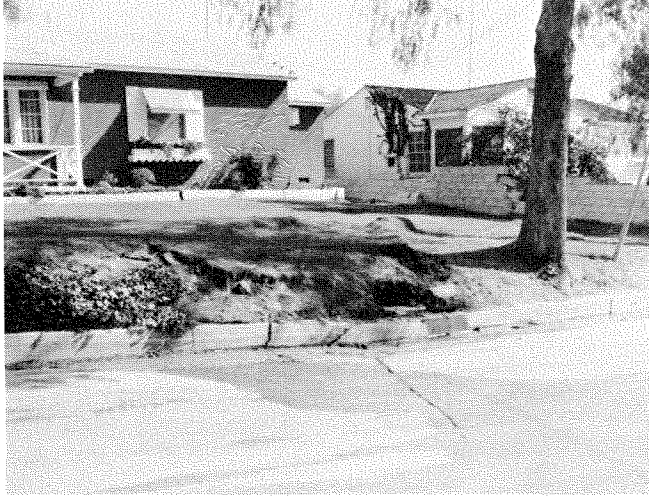
Photo 11. Fault displacement resulting from the San Fernando earthquake of February 9, 1971. Photo by James E. Kahle.
