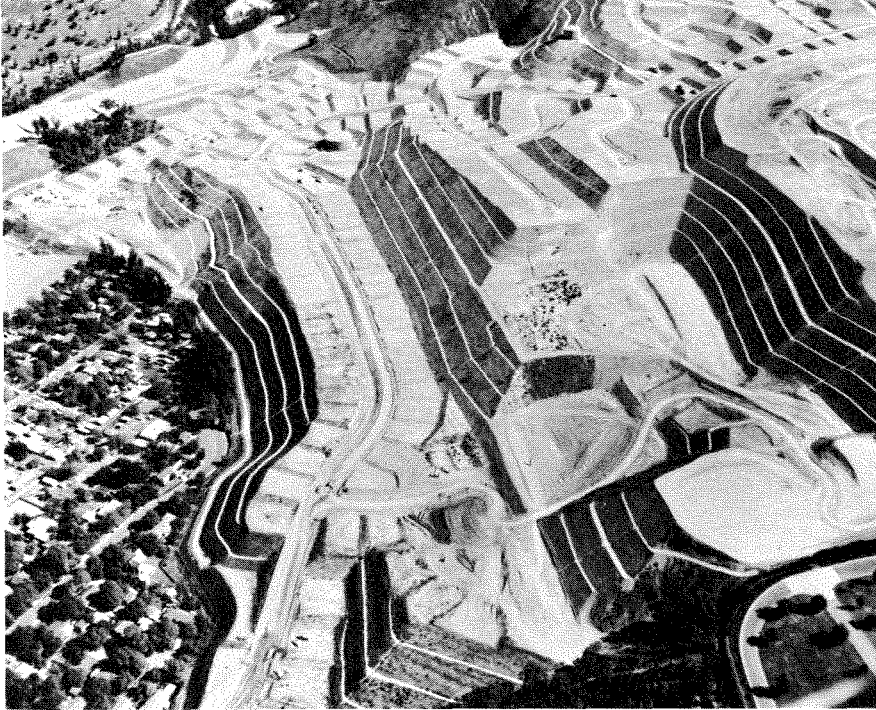
Photo 9. Erosion control measures used in a southern California subdivision. Narrow terraces and pipes are being used to bring water from the building sites safely down the hill. County of Los Angeles photo.
