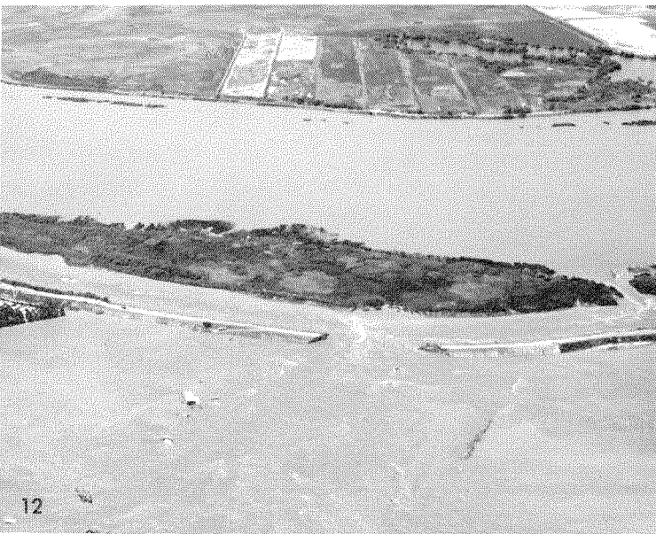
Andrus Island Levee Break
