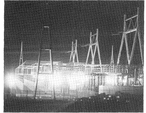
Switchyard at Oroville
