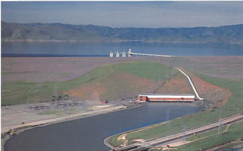
THE GIANELLI PUMPING-GENERATING PLANT (ABOVE) CAN BOTH PUMP WATER AND GENERATE ELECTRICITY WITH ITS EIGHT UNITS. SAN LUIS RESERVOIR (BELOW RIGHT), COMPLETED IN 1967, STORES 2,027,840 ACRE-FEET FOR STATE AND FEDERAL PROJECTS.
