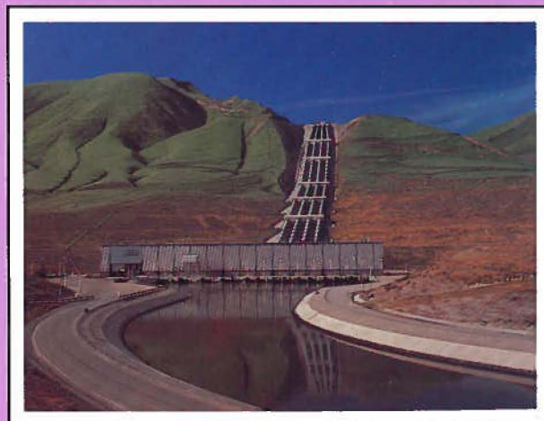
Chrisman Pumping Plant
