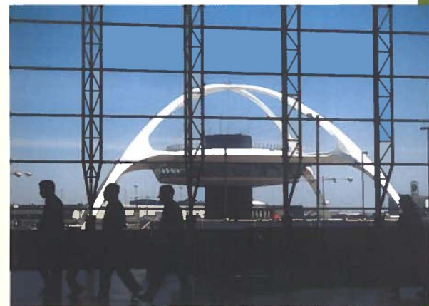
PHOTO CREDIT: LOS ANGELES INTERNATIONAL AIRPORT RESTAURANT, CALIFORNIA, L. BERKOWITZ/LOS ANGELES WORLD AIRPORTS
