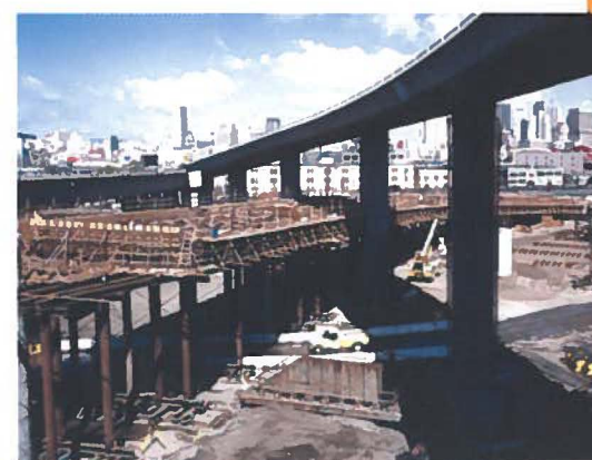
PHOTO CREDITS: TOP: TRAFFIC MANAGEMENT CENTER IN DISTRICT 7, LOS ANGELES, J. SPENCER/CALIFORNIA DEPARTMENT OF TRANSPORTATION BOTTOM: OAKLAND, CALIFORNIA DEPARTMENT OF TRANSPORTATION
