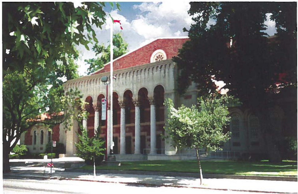
Sacramento Memorial Auditorium retrofitted for seismic safety, accessibility and energy efficiency, Sacramento, California
