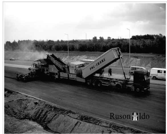
Fig. 1. Laying mineral asphalt mix in compact asphalt technology [7].
