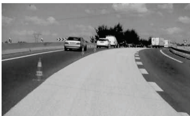
Fig. 8. Brightened asphalt pavement in Germany [6].
