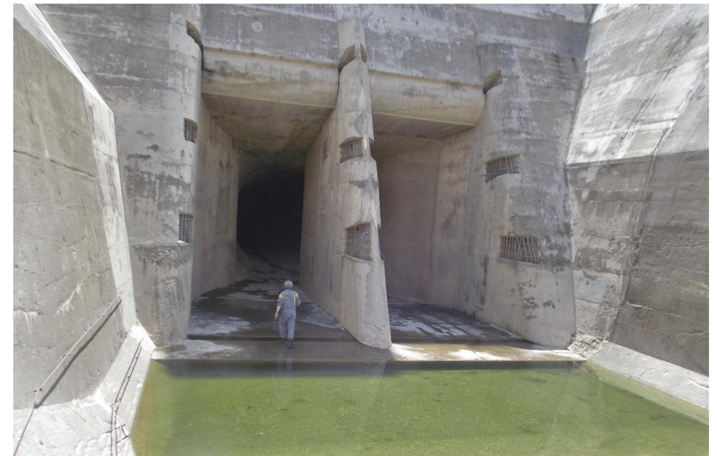
Figure 2. Entrance to the derivational tunnel
