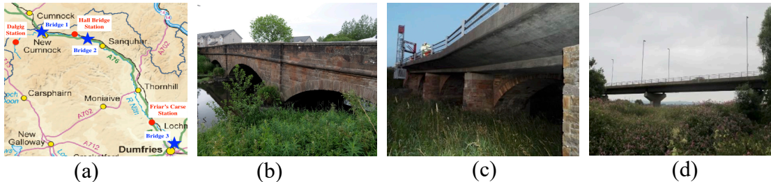
Figure 5: (a) Map; (b) A76 200 bridge; (c) A76 120 Guildhall bridge; and (d) A75 300 Dalscone bridge
