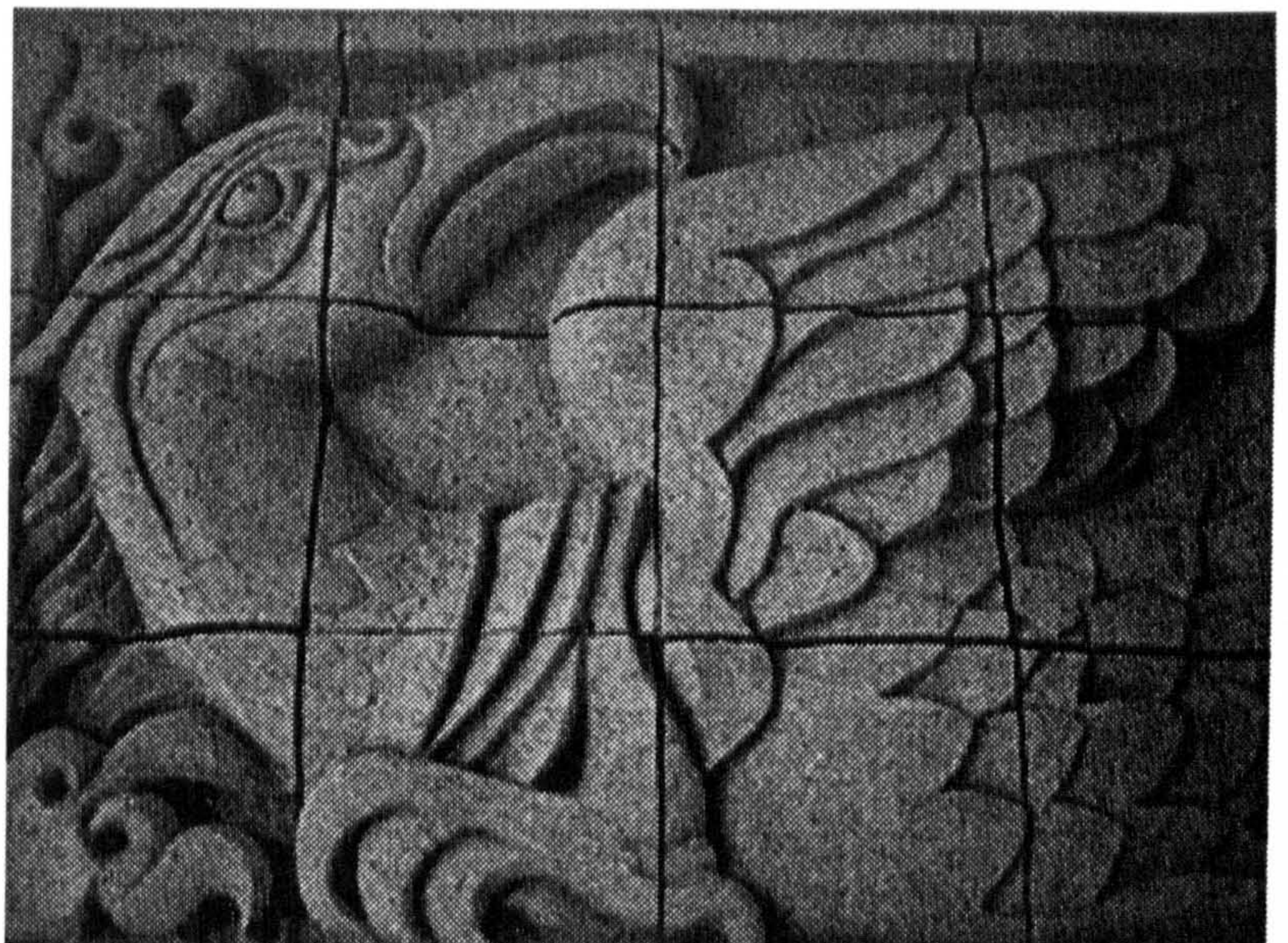
Detail, Carved brick panel
