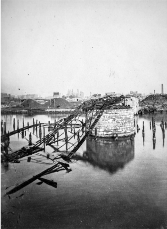
The Clark and Van Buren Street Bridge resting in the Chicago River following the fire.
