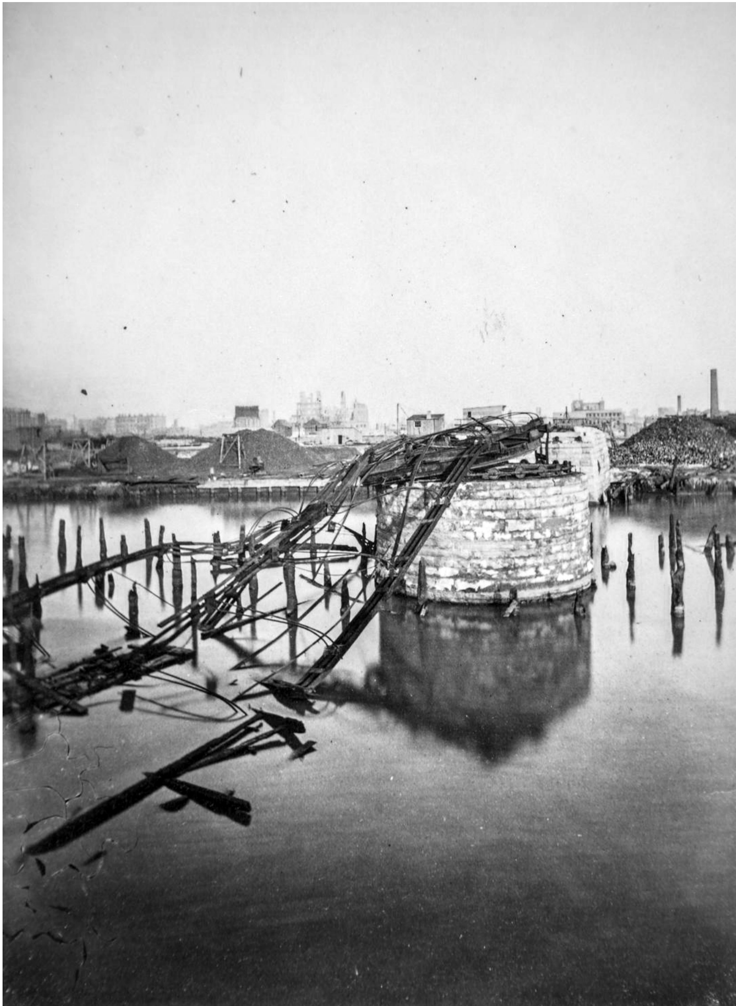
The Clark and Van Buren Street Bridge resting in the Chicago River following the fire.
