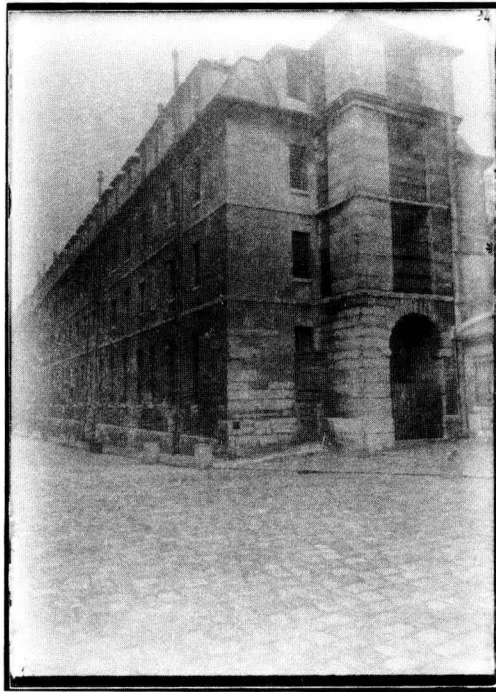
Exterior view of the prison wing.
