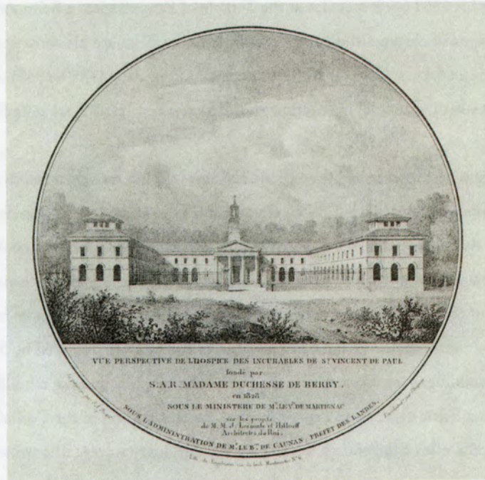
Figure 11: Jacques-Ignace Hittorff and Jean François Joseph Lecointe, Vue Perspective de L'Hospice des Incurables de St. Vincent de Paul , 1828, engraving. University and Municipal Library, Cologne (cat. no 12)
