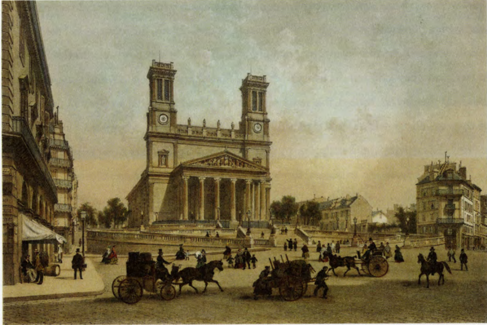
Figure 2: Felix Benoist and A. Bayot, Basilica of St. Vincent de Paul with a View of the Street , 1861, tinted lithograph. Special Collections and Archives, DePaul University Library (cat. no. 22)
