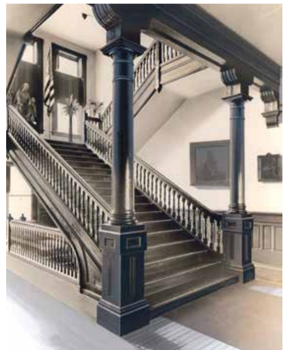
The circular main staircase constructed of oak.
