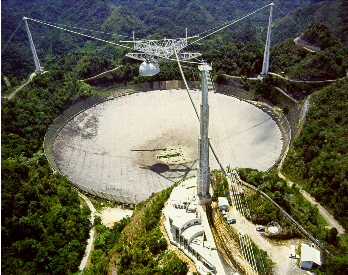
Figure 1.2: Photograph of the single dish Arecibo radio telescope (courtesy of the NAIC – Arecibo Observatory, a facility of the NSF). The Arecibo radio telescope is the largest single aperture telescope in the world, located in a basin in Puerto Rico with a diameter of 305 m (notice the cars in the lower right corner to appreciate the scale). Despite this large aperture size, due to the large wavelengths of radio waves, Arecibo still has a fairly poor resolution ( 0.5' in X-Band 12–18 GHz to 3.5' in L-Band 1–2 GHz), making it a poor imaging instrument. The large collecting area does make it an ideal survey instrument, as Arecibo is then able to observe large portions of the sky in a small amount of time.
