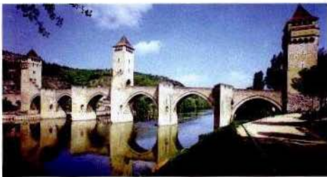
Valentré bridge over the Lot, Cahors
