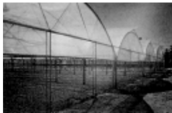
Fig. 12. Tunnel-shaped greenhouses covered with double EVA film.
