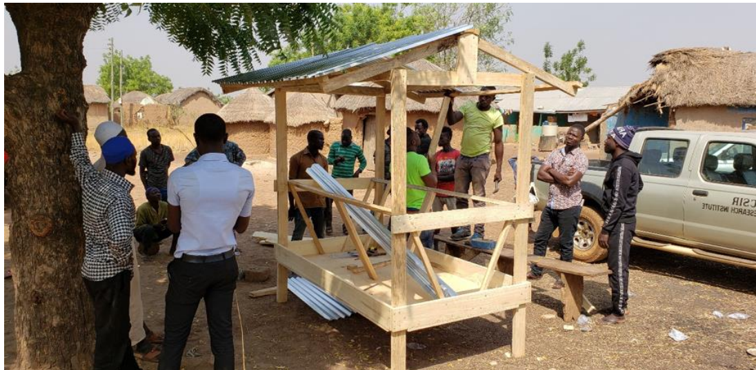
Picture 1: Members of Youth Empowerment for Life (YEfL) and farmers observing construction of feed trough in Tibali. Photo credit: Sadat Salifu/CSIR-ARI.
