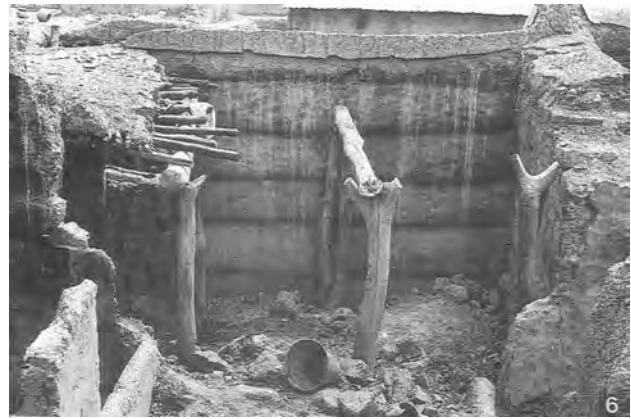
Fig. 2 Construction area with pisé and mudbrick wall (Schneider 1991 Photo 6).
