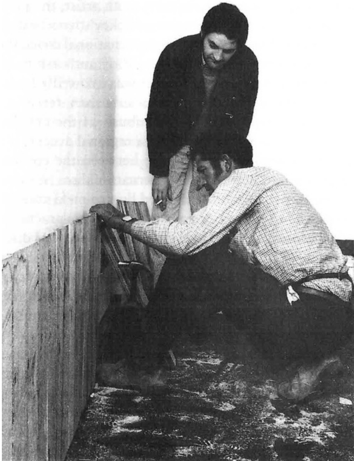
Figure 3.2: Dale Hickey and fence-builder Jim Emmins, during the installation of Fences , 1969.
