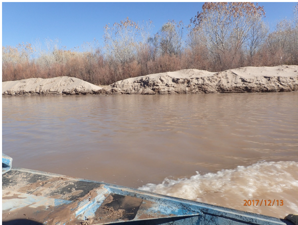
Photo 10: Looking east at spoil berm from 2017 pilot channel through the sediment plug. Spoil piles are actively eroding (Holste, December 2017).
