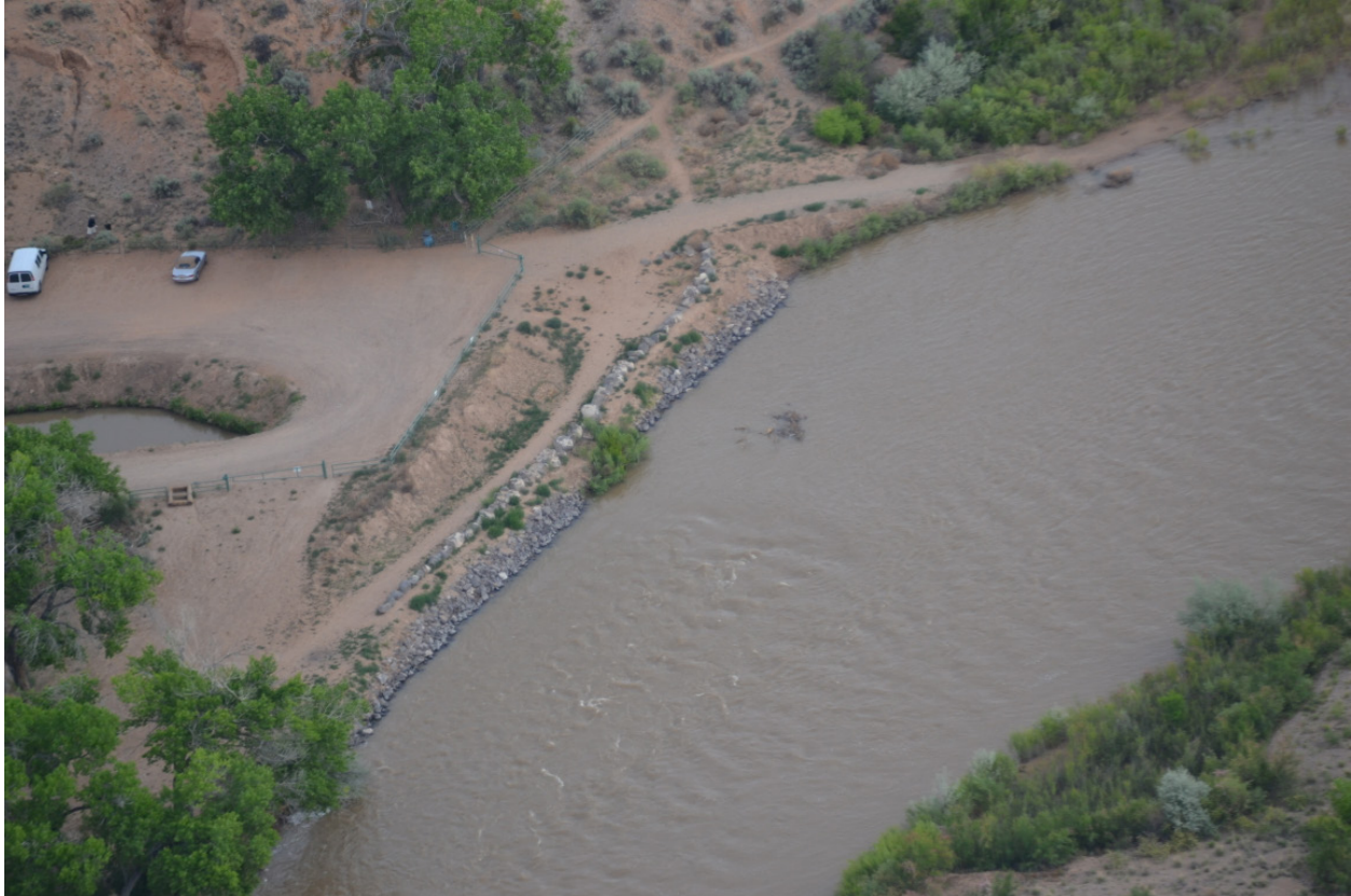
Photo 5: Aerial view of Corrales Siphon (Padilla, May 2017)
