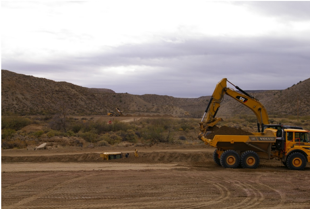
Photo 11: Relocation of previously stockpiled sediment (foreground) away from active arroyo (background), looking up Mescal Arroyo near Rio Grande confluence (Harris, December 2017)
