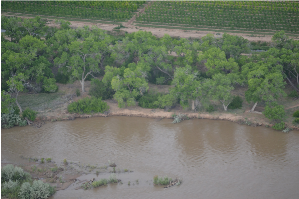
Photo 6: Bank erosion at River Mile 199 (Padilla, May 2017)
