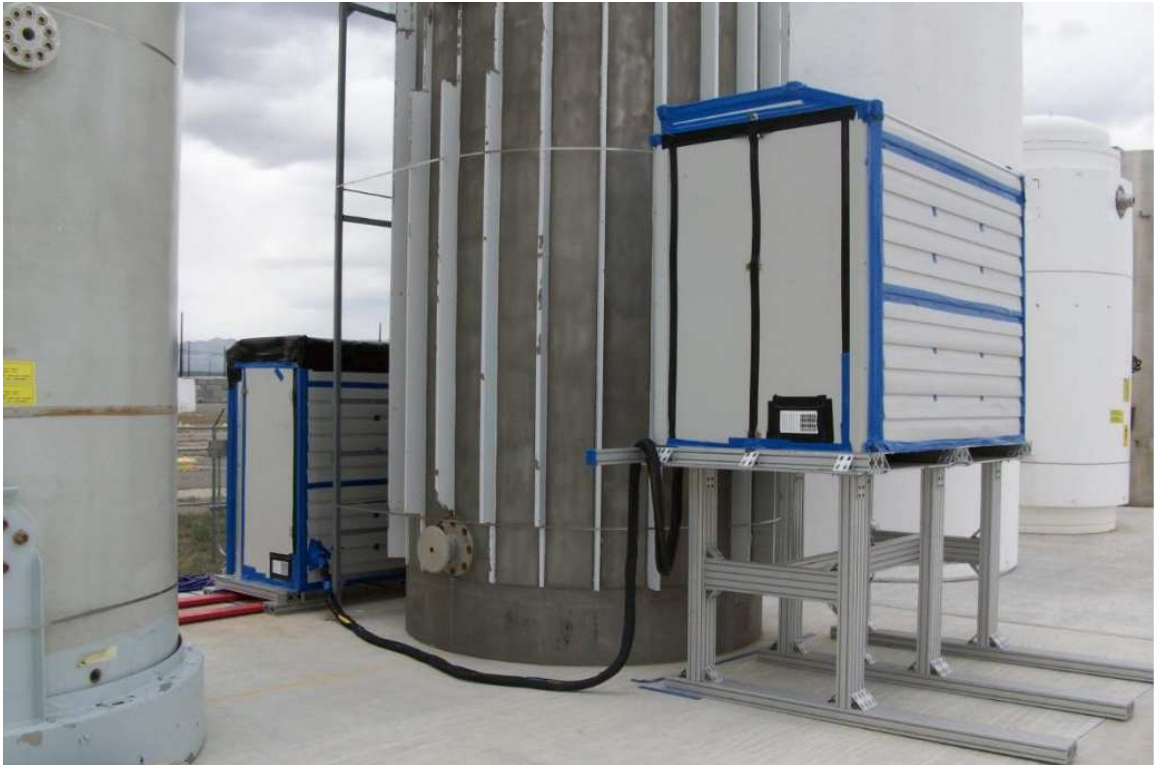
Figure 4.8: Two weatherproof enclosures, each containing 1 supermodule. The near supermodule is elevated to increase the muon flux and decrease the counting time.
