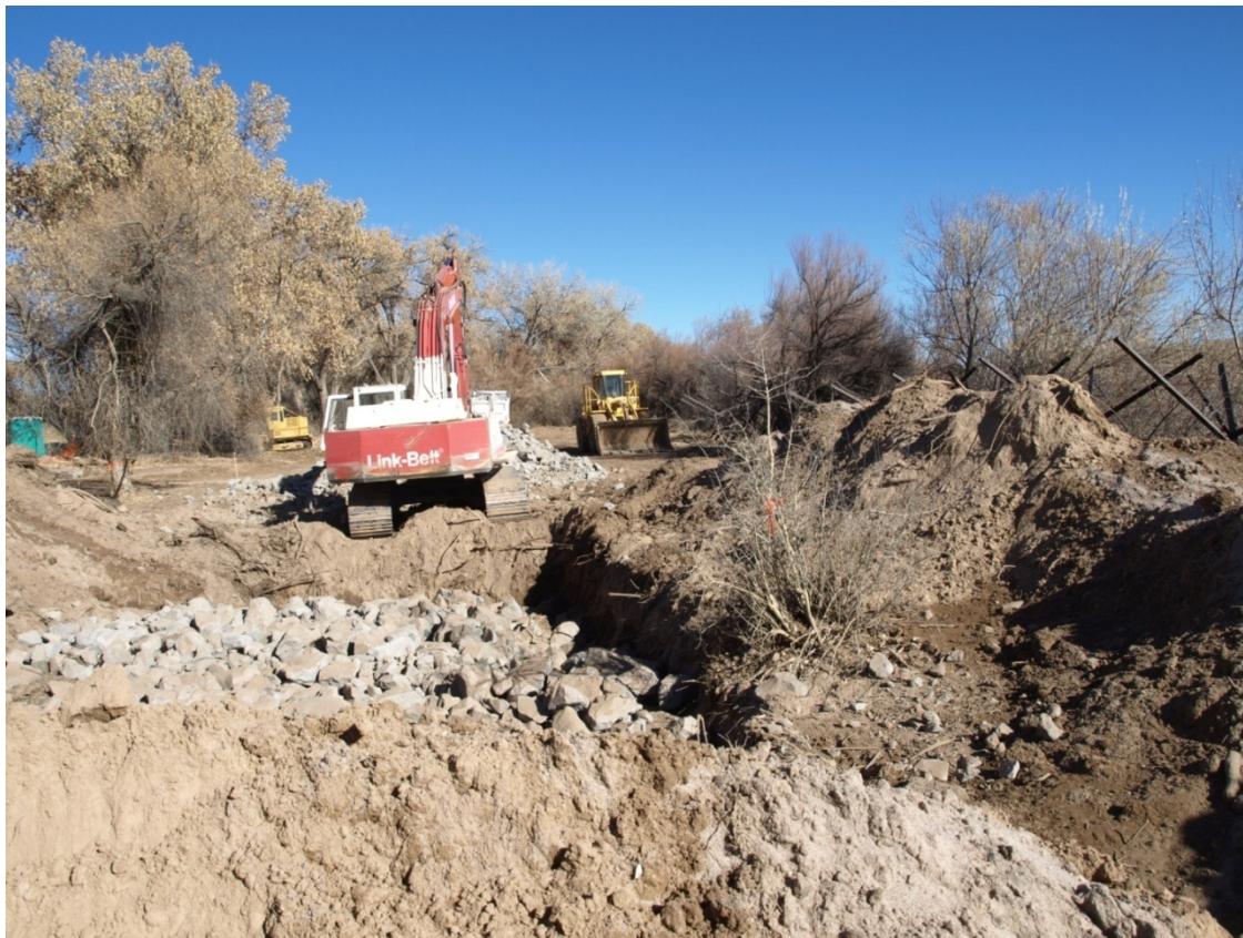
Photo 5: Santo Domingo Pueblo RM 225.1, placing self launching riprap (December 2012, AuBuchon)
