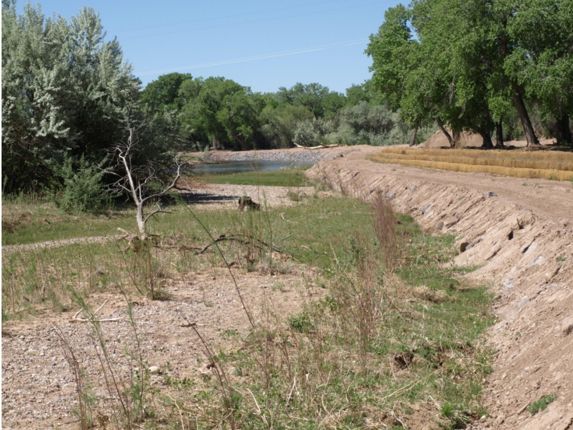
Photo 6: Coyote willow whips, rock toe, and Bio-D blocks at Priority Site RM 212.0 (May 2012, Walton)
