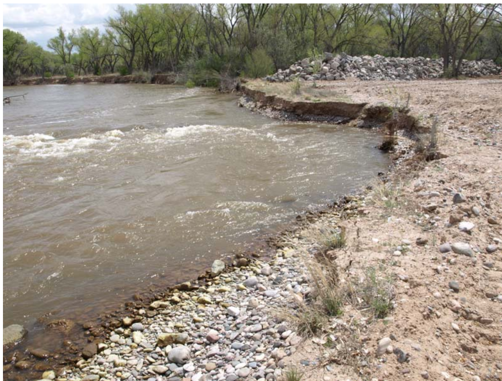
Photo 5: San Ildefonso bankline erosion and riprap windrow (May 2010, Holste)
