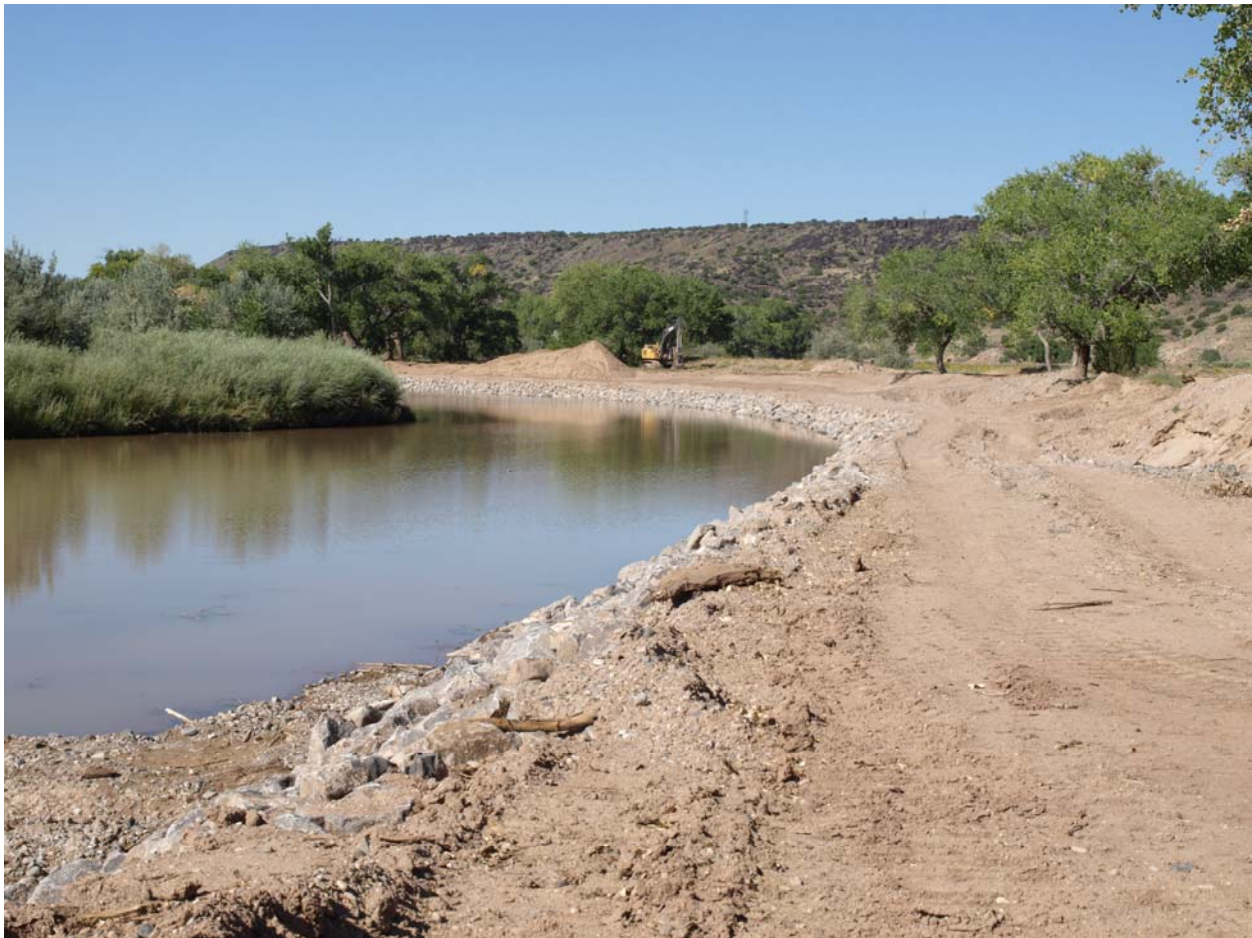
Photo 8: Rock toe placement at Priority Site 213.4, San Felipe (September 2010, AuBuchon)
