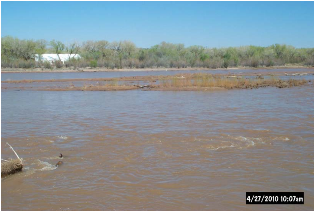
Photo 11: Increased wetted width at higher flows (approximate river flow is 2800 cfs) from the Corps of Engineers' bar lowering at the Pueblo of Santa Ana across from the Santa Ana RM 205.8 priority site (April 2010, AuBuchon)
