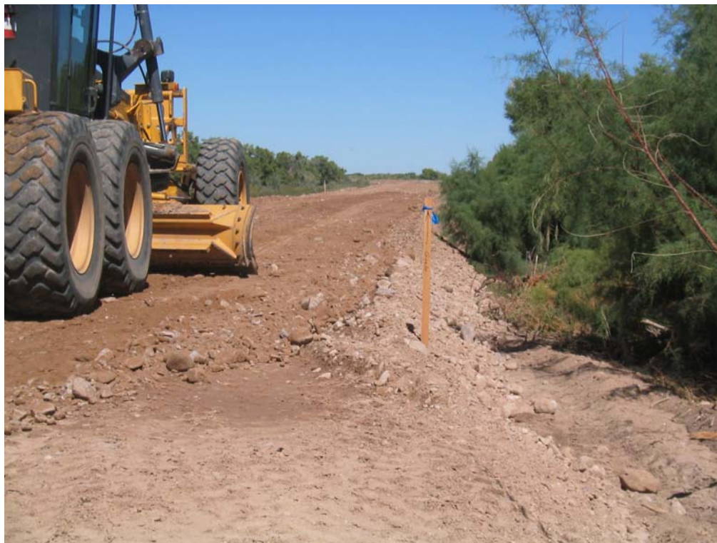
Photo 16: Levee raising north of BDANWR (September 2010, Weems)
