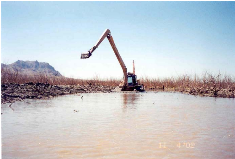
Figure 6: Downstream view of an Amphibious Excavator working in the Temporary Channel (4/2002)
