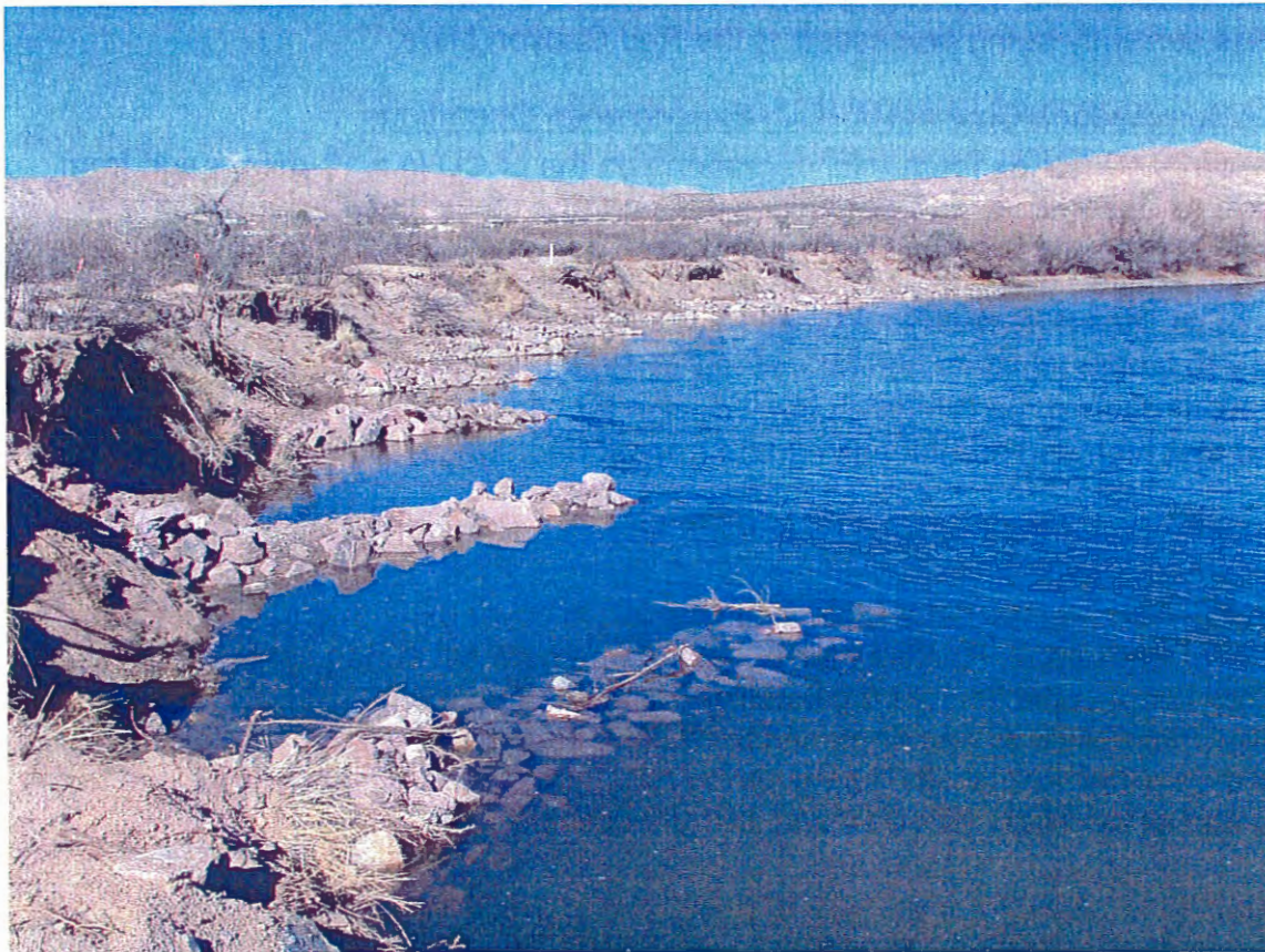
Photo 8: Bendway weirs installed near Williamsburg Bend.
