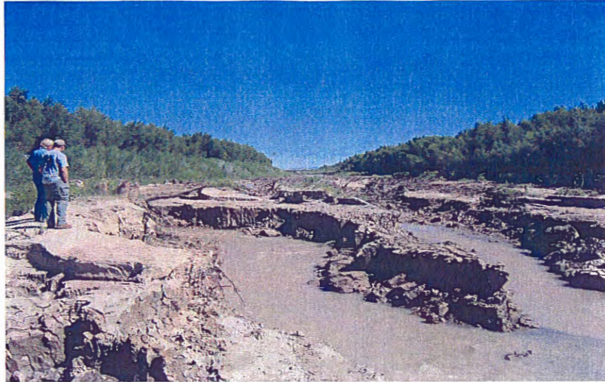
Photo 2: Temporary Channel 2000 headcutting (2004)
