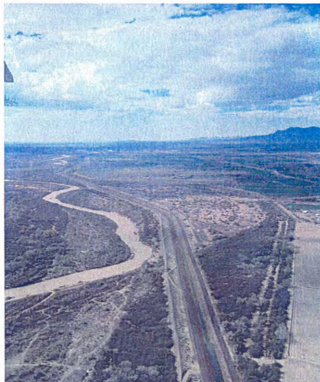
Photo 7: Looking downstream at RM 114 and 113 Levee Setback Project. Levee and LFCC will be moved to the west (right).
