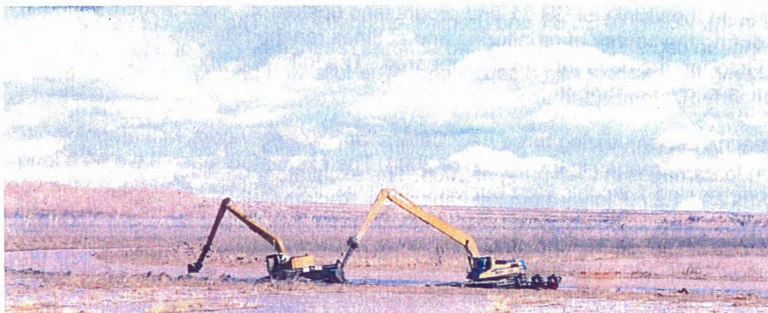
Photo 3: Temporary Channel 2002 excavation.
