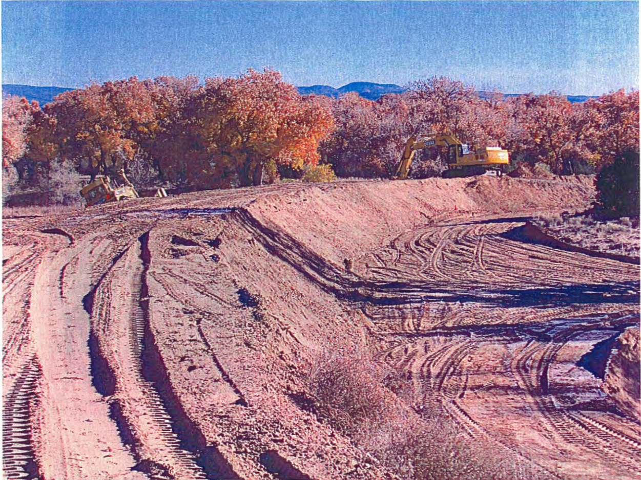
Photo 6: Construction at the Santa Fe River confluence.
