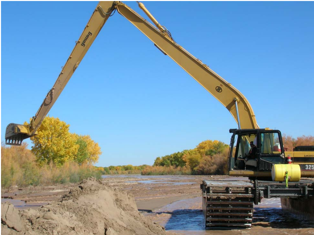
Photo 20: Pilot channel excavation at the Tiffany Sediment Plug, November 2005
