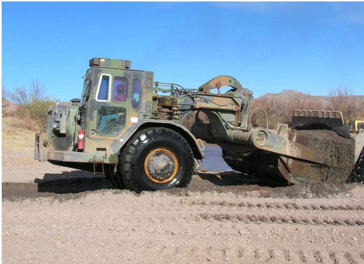
Photo 21: Removal of sediment at the Arroyo Hondo confluence near Truth or Consequences, December 2005
