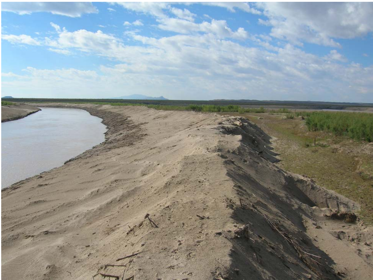
Photo 4: Excavated channel and berm downstream of the Narrows, October 2005
