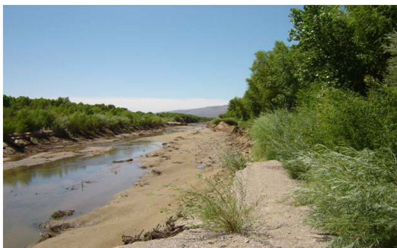
Photo 2: Looking south at washout around EB-26 on the Temporary Channel access road (2005)
