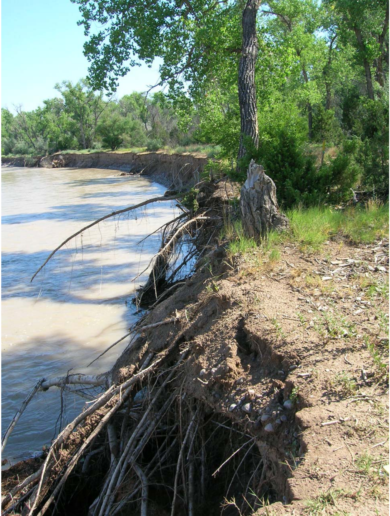
Photo 8: Bank erosion upstream of the San Ildefonso Pond, July 2005
