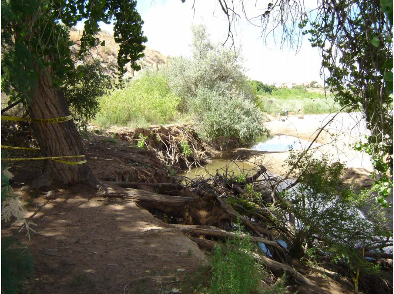
Photo 29: Post Runoff review at the Corrales Siphon location looking upstream on west bank showing bank erosion underneath large cottonwood tree (July 2005)
