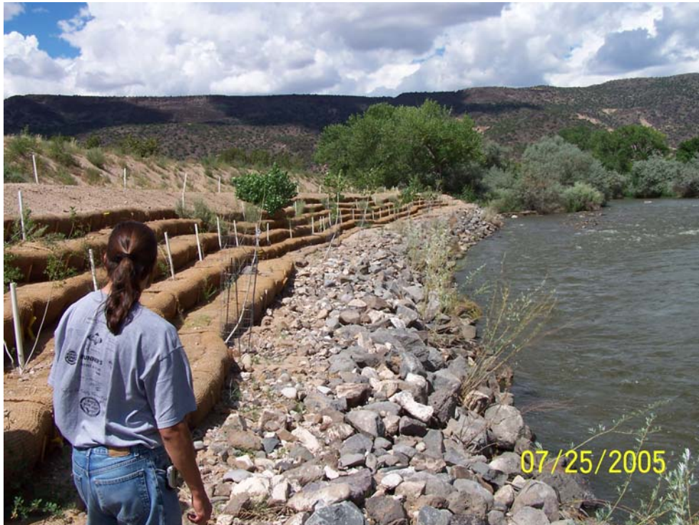
Photo 6: Looking upstream at the La Canova site after runoff (July 2005)
