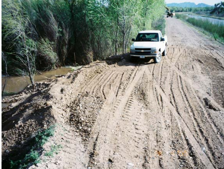
Photo 28: San Marcial Levee near Ft. Craig showing completed repair work (2005)
