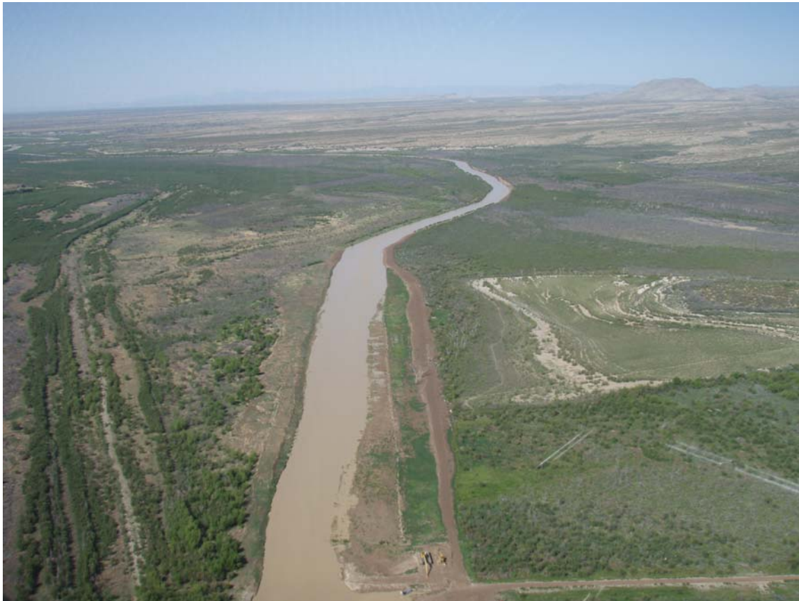
Photo 2. Temporary Channel 2000 to 2002 transition. Taken near RM 52, facing downstream (May 2007).
