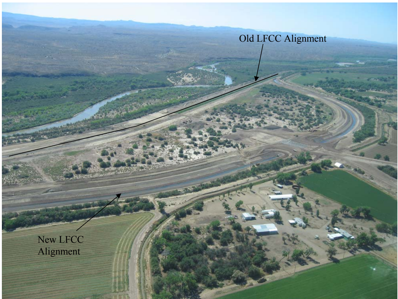
Photo 10. Looking downstream at the new LFCC in the area of River Mile 113/114 Priority Site (May 2006)
