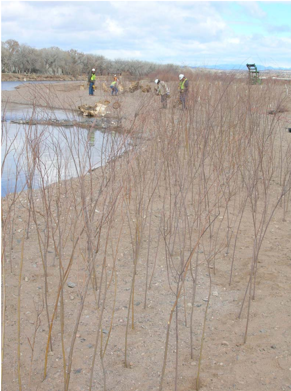
Photo 7. Installation of native vegetation at the Bernalillo priority site (February 2007).
