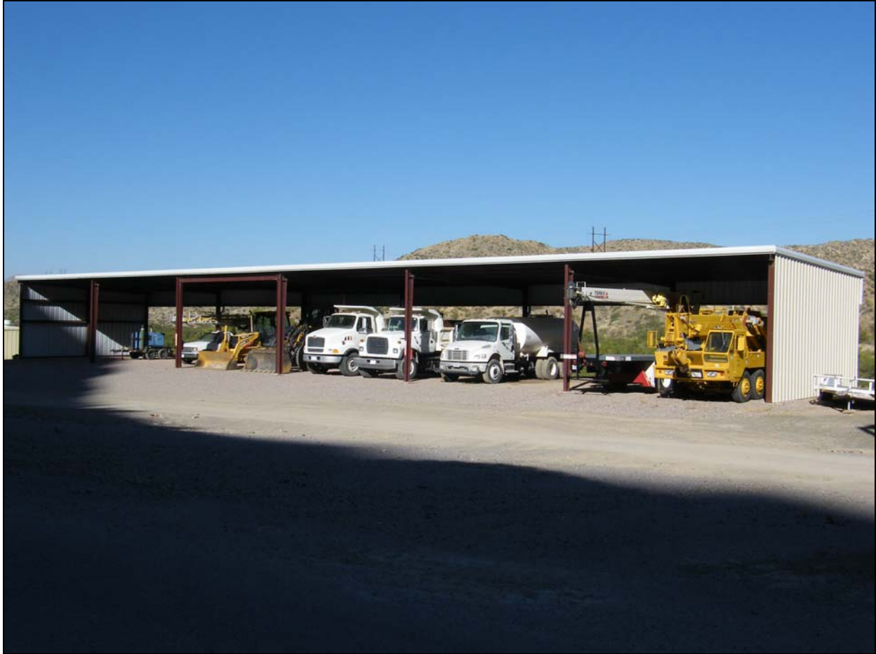
Photo 27 - New equipment cover at Elephant Butte Dam yard.
