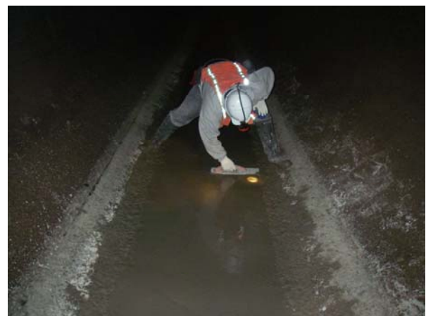
Photo 2. Azotea Tunnel after repair
