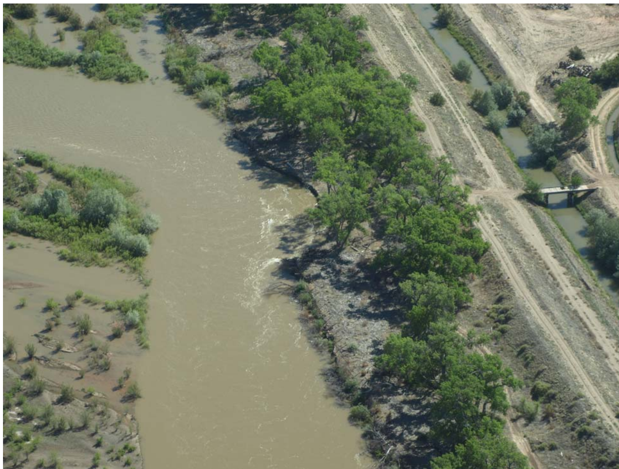
Photo 15. Aerial view looking upstream toward the bend erosion at the Santa Ana Tamaya site (June 2008, Padilla)
