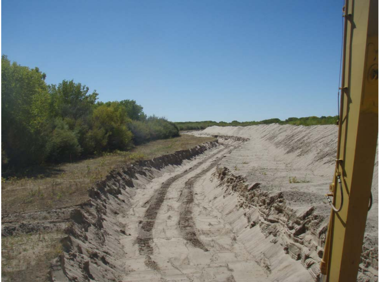
Photo 22. Bosque del Apache pilot channel excavation, looking downstream (October 2008, Rolland).
