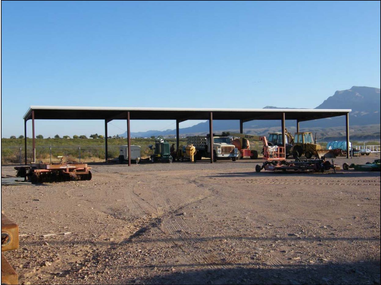
Photo 26 - New equipment cover at the Caballo Dam yard.
