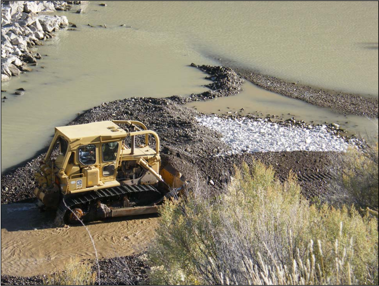
Photo 35 - River work near the tailbay to the Elephant Butte Dam.
