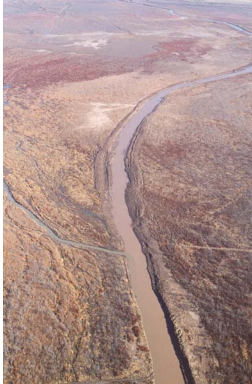
Figure 6: Upstream view of the confluence of LFCC spillage and the Temporary Channel (1/2003)
