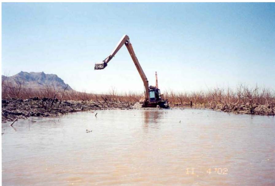
Figure 7: Downstream view of an Amphibious Excavator working in the Temporary Channel (4/2002)
