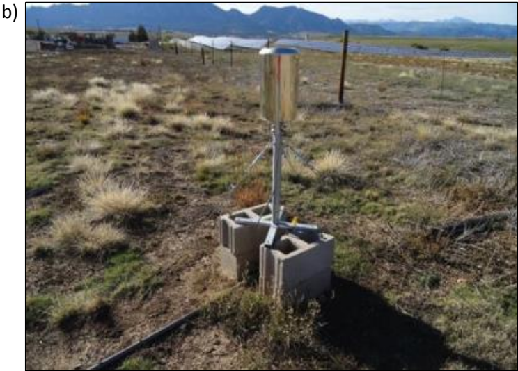
Figure 1: Thies Precipitation Transmitter installation at (a) Formigal and (b) Marshall.
