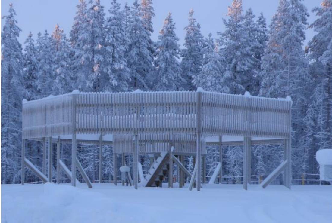
Figure 3.8. Field working reference system R2, as configured on the Sodankylä SPICE site, Finland.
