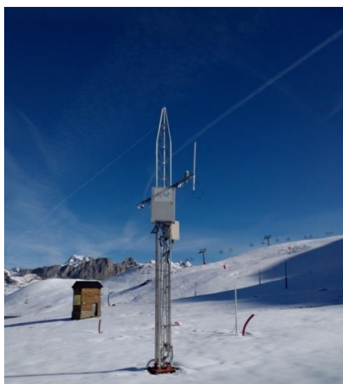
Figure 4.79. Installation of the SR50A sensor at the Formigal site.
