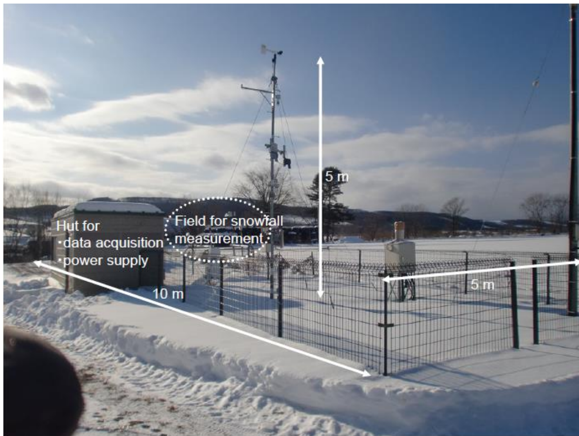
Figure 1. Overview of Rikubetsu SPICE site
