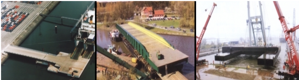
Photograph 8: Ro-Ro ferry facilities – linkspan and pontoon
