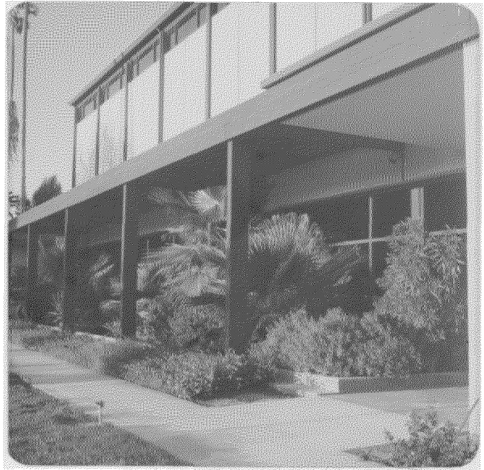
Fig. 50. Gardens along the side of the Riverside Church. The clear glass windows separate the outdoor gardens from the planters inside. The effect is one of a "total natural" setting for worship.
