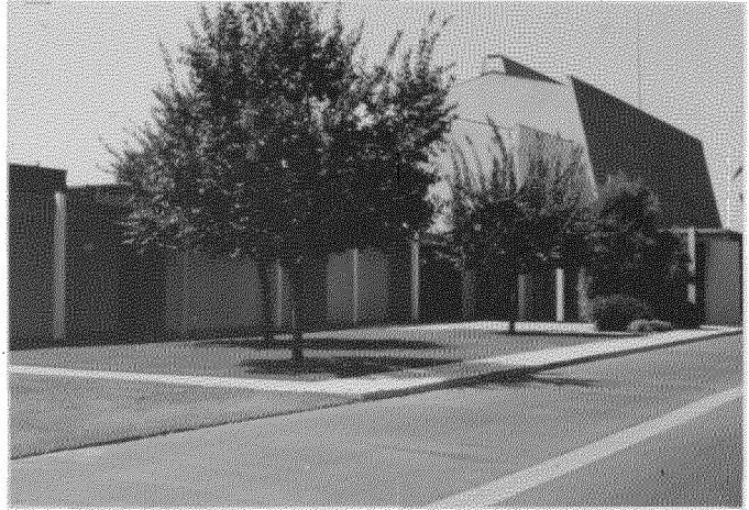
Fig. 32. The Anaheim Church, viewed from the side rear, showing the open breezeways of the classroom area.
