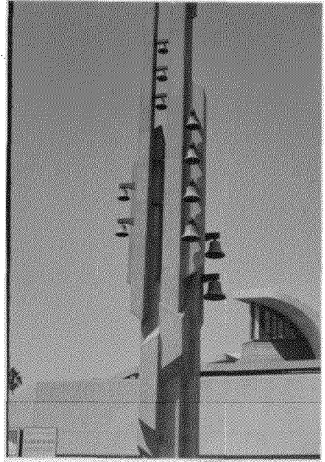
Fig. 48. The controversial new Presbyterian church, Pasadena. It is highly innovative but also very expensive
