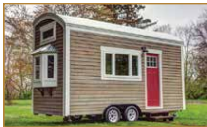
School of Architecture, Art & Design students at Andrews University built two tiny, completely livable houses on 18-foot trailers.
