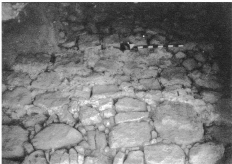
Figure 7. Tall al-'Umayri, Field A (Phase 13): Elevation of the early Iron I perimeter wall; note plaster remnants in cracks.
