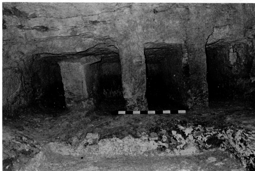
2. Interior view: north wall.
