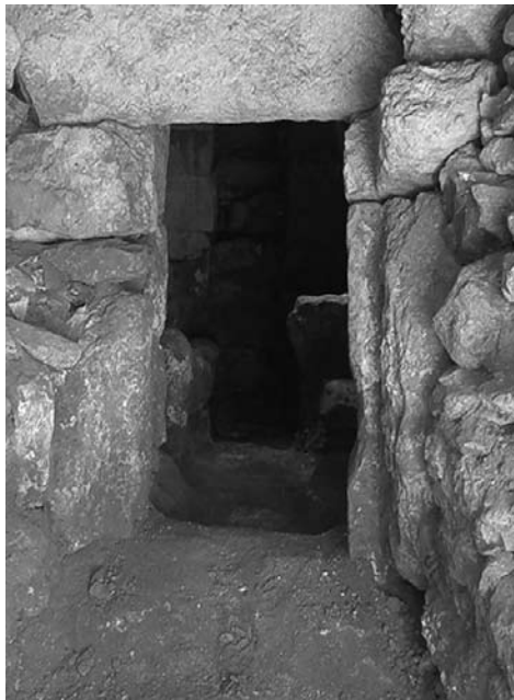
Figure 28. Door to the granary in lower-level of the two-story building in JIV Square.
