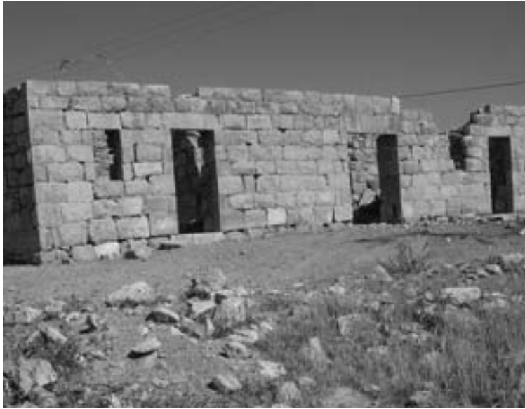
Figure 35. Building 5 in the JIV.
