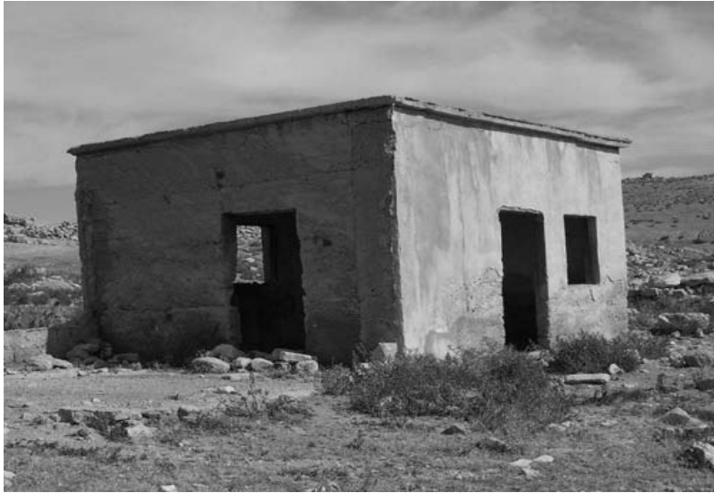
Figure 33. Building 1 in the JIV.
