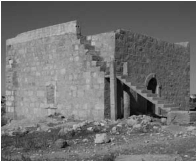
Figure 34. Building 3 in the JIV.
