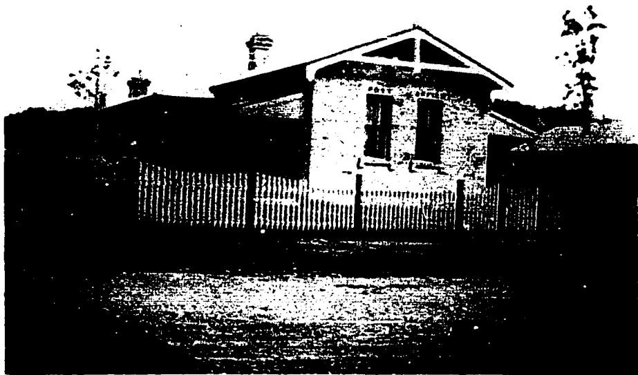
Fig. 25. Cooranbong post office
