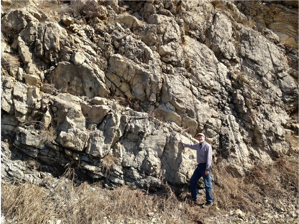
TEXT-FIGURE 19.—Folding in the Fort Sill Limestone, stop 10 (GPS: 34°24'29.76"N, 97° 8'20.85"W).
