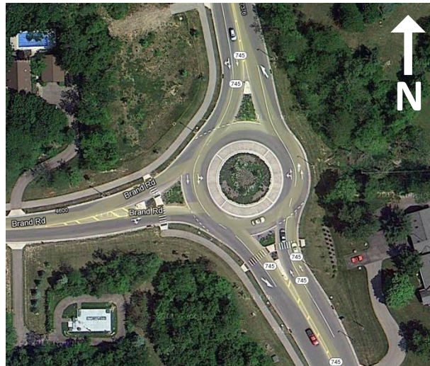
Figure 6 – Brand Rd and Dublin Rd Roundabout
