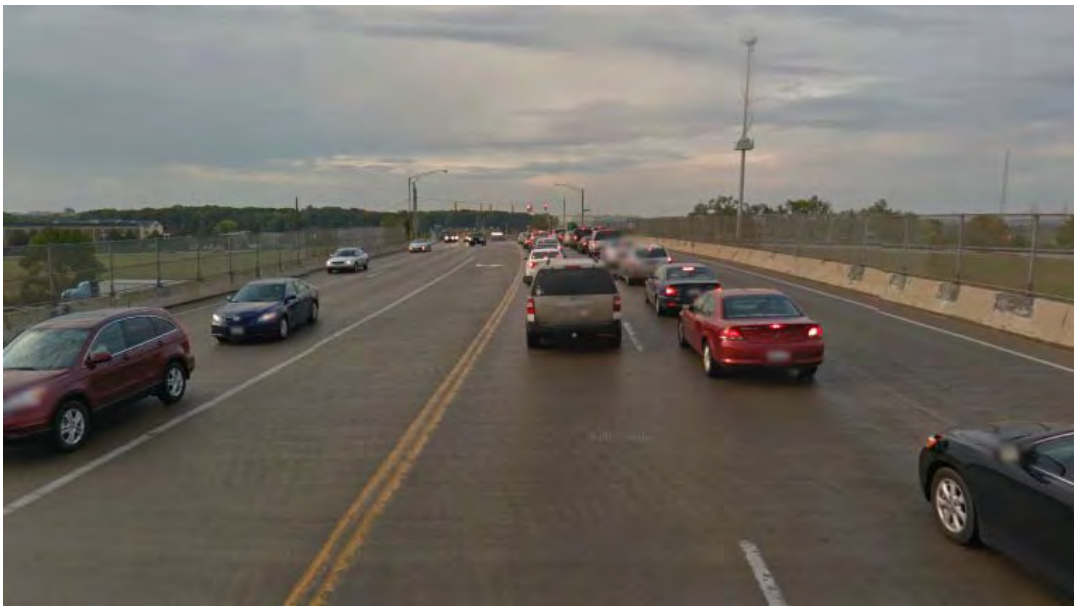
Figure 12: North Fairfield Road Overpassing I-675.
