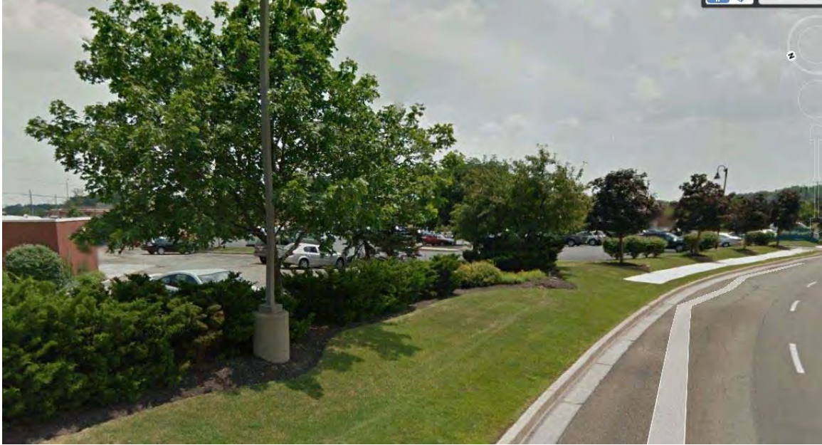
Figure 15: Unconnected Sidewalk along Ring Road at the Mall at Fairfield Commons
