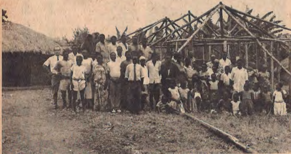
MEMBERS of the Baptist congregation in the rural village of Bumbo, Uganda, stand in front of the framework of what is to be their new church building. The original thatch-roofed structure is at left. After the Sunday morning service, members of the East African church walked a mile to a stream for baptismal services. Southern Baptist Missionary Jimmie D. Hooten (left) baptized the converts. (Photo by H. Cornell Goerner)
