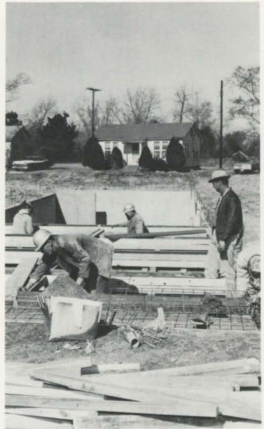
Construction of the new gym gets well under way with Gary Stephens, Leroy French, and other members of the campus crew doing the construction.
