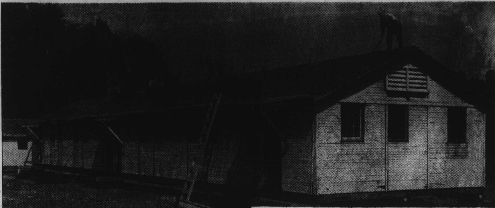
Under the eager, and in some cases startled gaze of students and faculty, the wood-piles on the campus take shape. It is hoped they will be completed by the first of next month.
