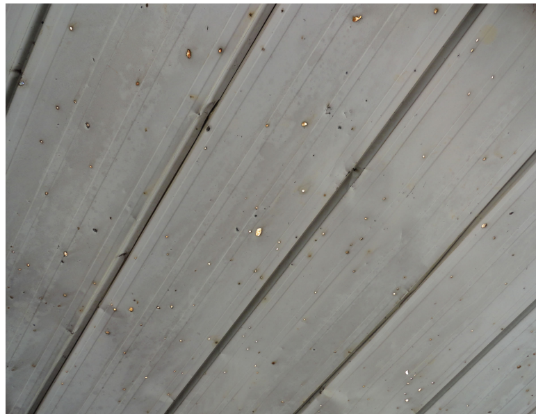
Figure 8A and 8B: Damage from grenade and artillery fire.
