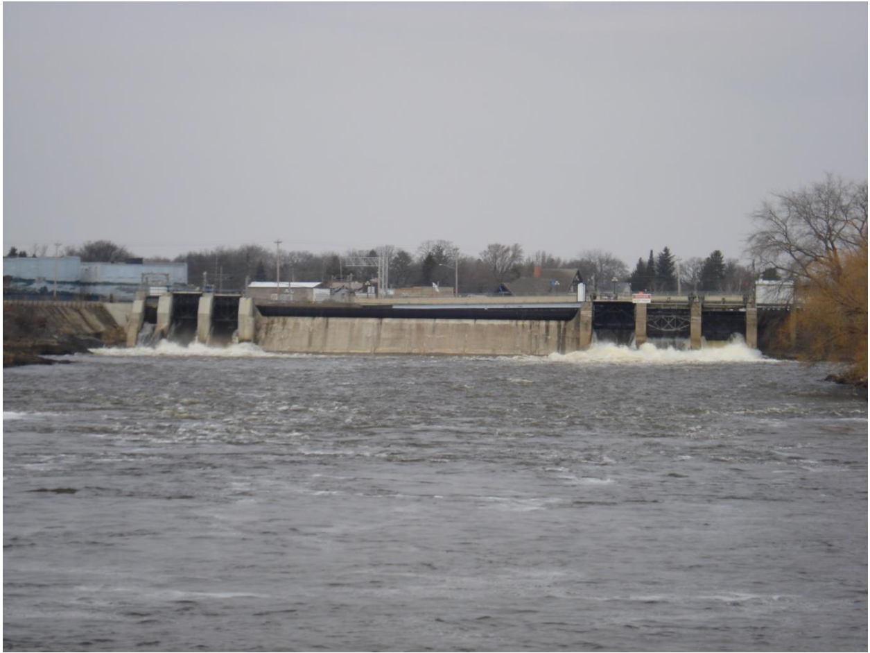
Figure 3: Little Falls dam as seen from downstream.
