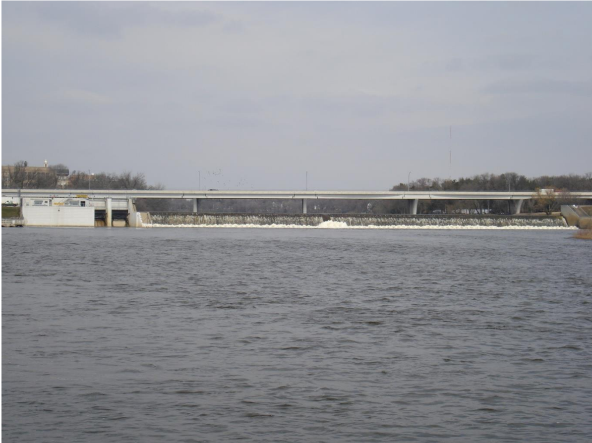
Figure 9: St. Cloud Dam as seen from downstream.
