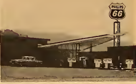
The new College Service Center has five green racks, a wash rack and motor car sections. It has the latest in all facilities.
