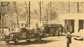
Preparing to do battle, the department's two trucks load men and equipment on Apison Pike. Calls to the station result in the activation of the volunteerspower siren atop the administration building.
